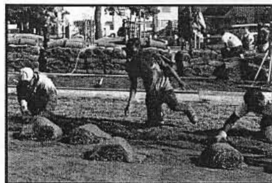
Laying sod at the Sunnydale Community Center ▲
